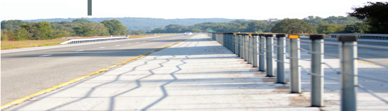
Indian Nation Turnpike Positive Barrier Installation
