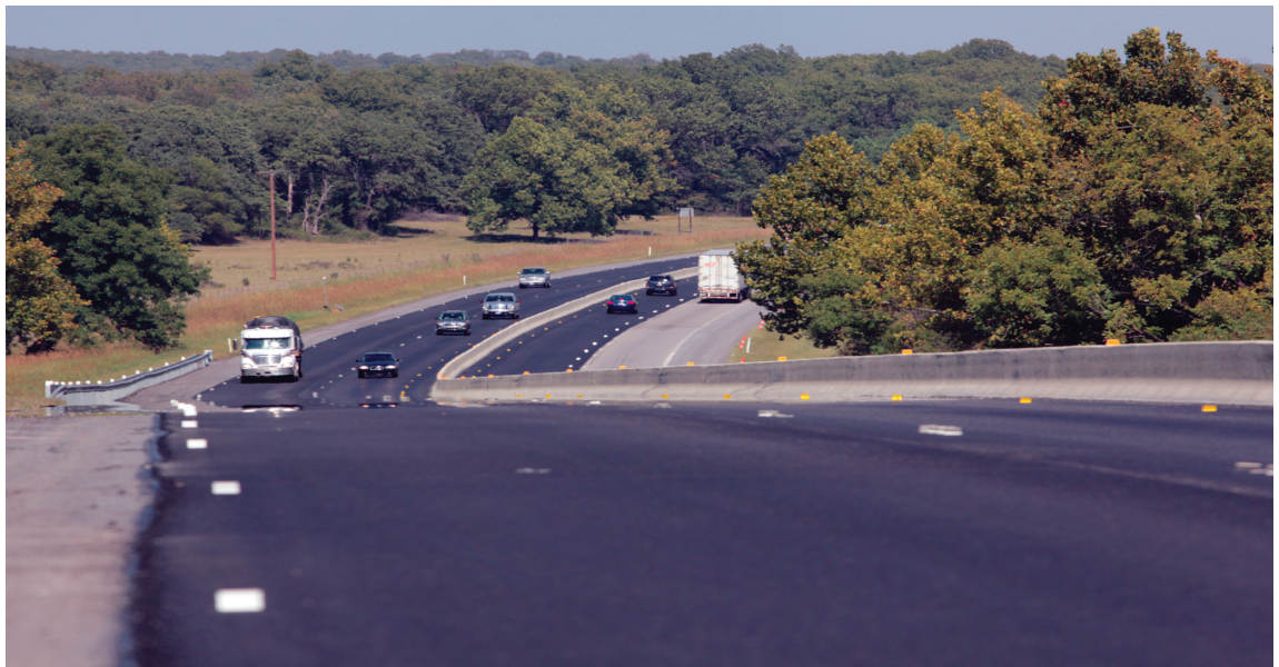
Turner Turnpike Pavement Rehabilitation
