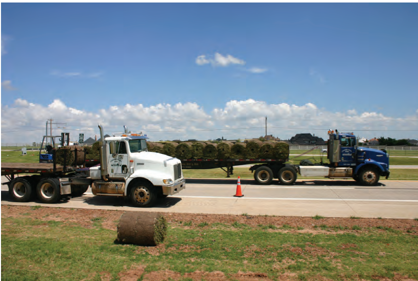
John Kilpatrick Turnpike Laying Sod
