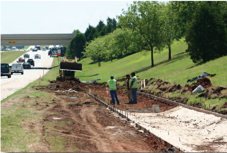
John Kilpatrick Turnpike Drainage Project
