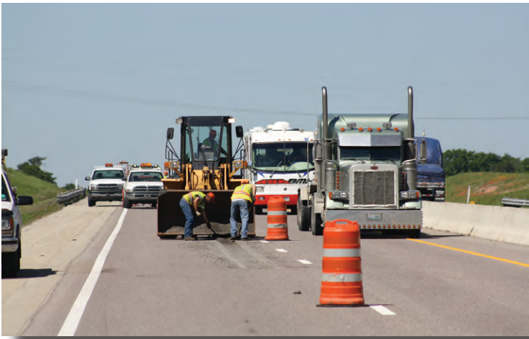
Turner Turnpike Laying Asphalt
