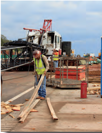
Turner Turnpike Bridge Replacement
