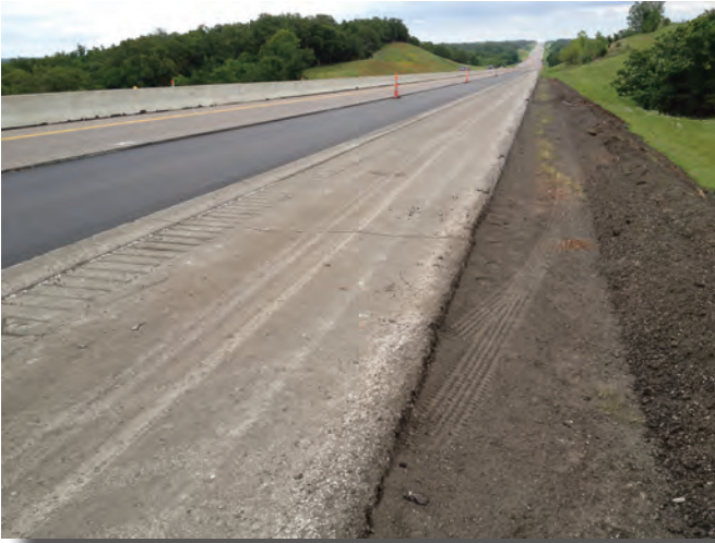
Turner Turnpike Pavement Rehabilitation
