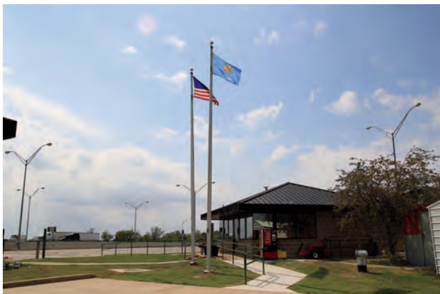
Turner Turnpike Toll Plaza Electrical Upgrade
