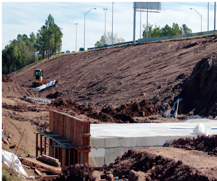
Creek Turnpike Interchange Improvements at Elm Street
