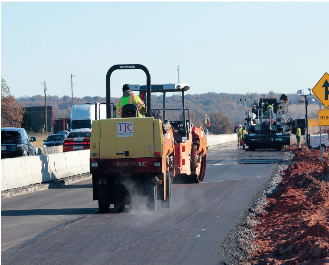
Turner Turnpike Wellston Interchange Pavement Rehabilitation
