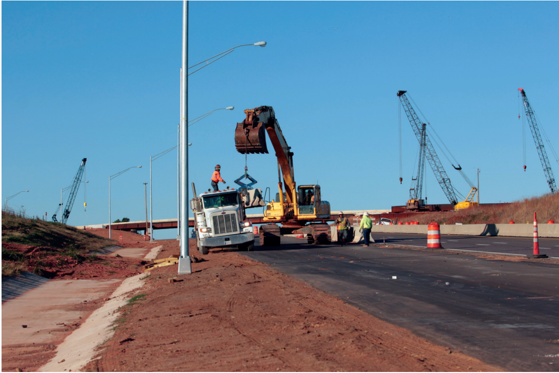
Turner Turnpike Luther Interchange Bridge Replacement
