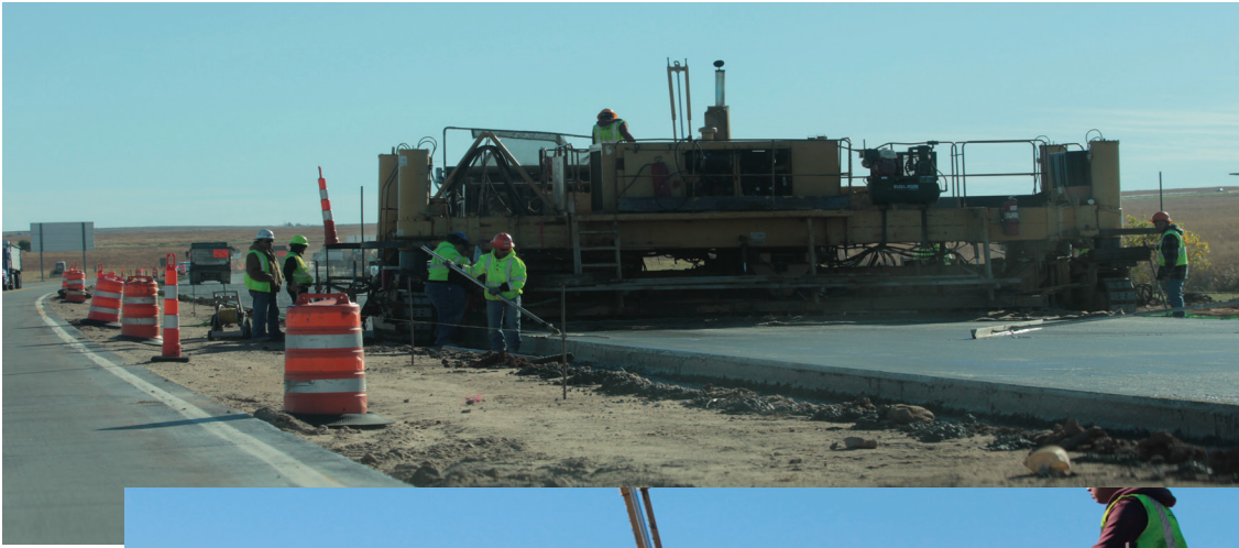
Cimarron Turnpike Pavement Replacement
