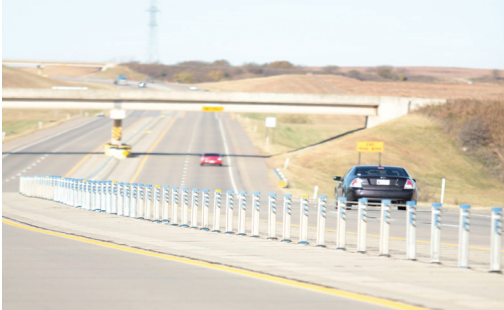
Cimarron Turnpike Positive Median Barrier
